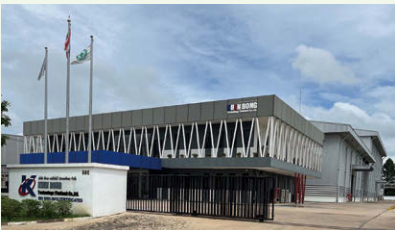
Kuen Bong Technology (Thailand) Co., Ltd.
