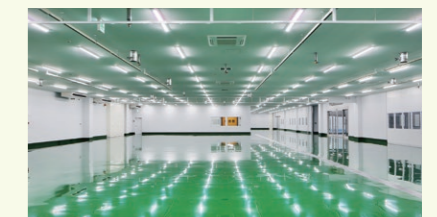
Installation image of Fabbrica Floor Coating SCR Method
