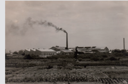
High-pressure laminate (HPL) plant completed in 1959
