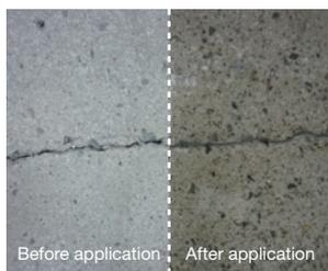
Clear membrane makes it possible to check changes in the crack after application
