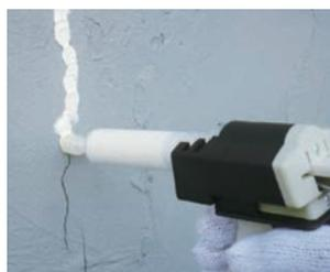
Gun-type applicator enables quick and easy repairs of cracks in concrete
