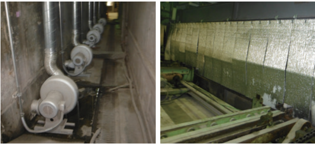
Air distribution fan (left) and heat retention curtain (right) newly installed to stabilize temperature inside curing chamber
