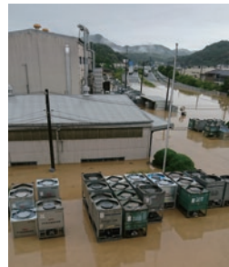
Photo taken July 7, 2018 Flooding
